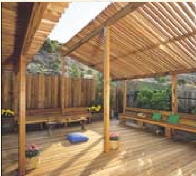
Deck and angular trellis addition. A Construction Common deck is enhanced by a shady set of twin trellises with a sloping design. Built-in benches and redwood fence complete the attractive setting.
