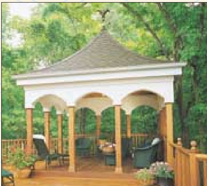
Pagoda deck shelter. Construction Heart deck is enhanced by a pagoda-like gazebo. The structure is characterized by eye-catching curves and arches and includes a ceiling fan and antique weathervane.
