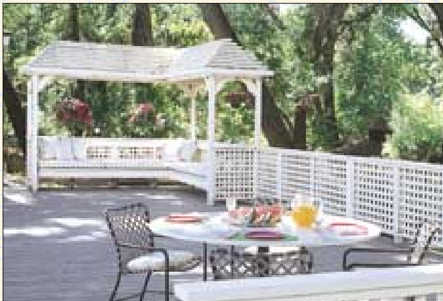
Corner bench deck shelter. L-shaped bench transforms a bare corner of a deck. The 9x9 structure has a hip roof that creates a shady retreat. Classic redwood lattice panels form the back of the bench, echoing adjacent deck railings.
