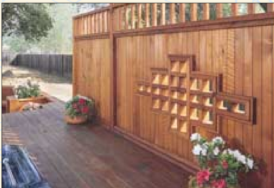
Eye-catching privacy screen. Part of an overall redwood deck project, a Construction Heart/Deck Heart fence shields a spa setting from neighboring yard. The intriguing design includes sculptural cutouts and top trim of redwood uprights.
