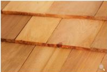
Cedar shake roof
