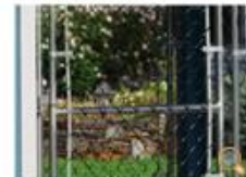
Vinyl Coated chain-link fence
