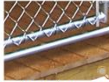
Composite decking on run area
